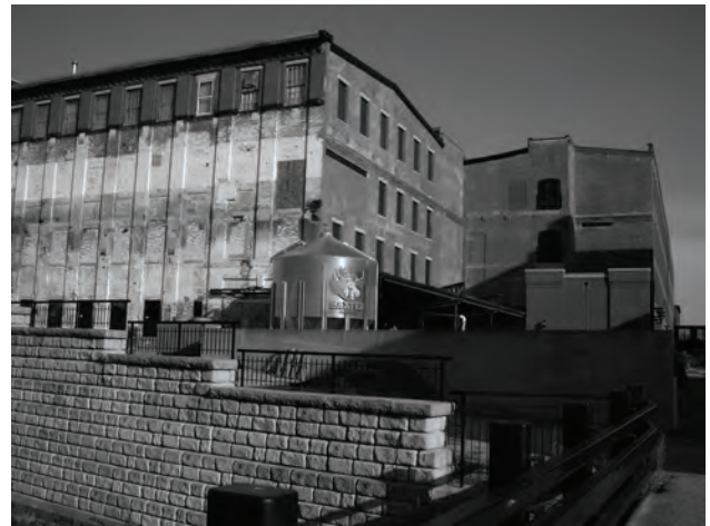
Wing House # 1 used as a Picker House, houses Baxter Brewery
