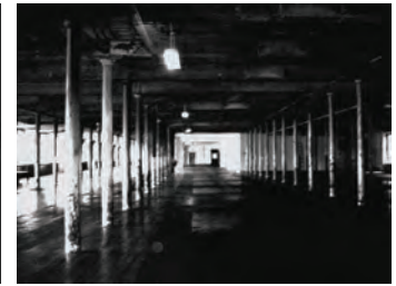
Inside of Mill # 1, Round Columns are made of wood.
