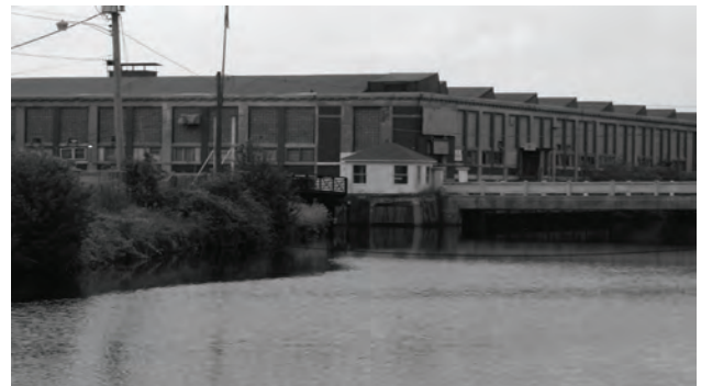
Canal side of # 5
