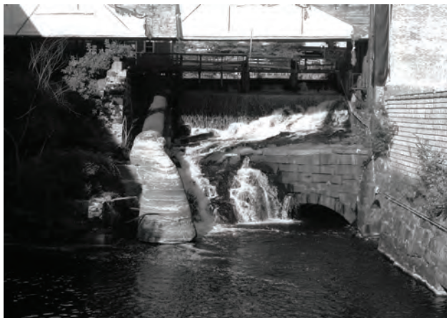
Same walkway showing Canal with falls under the walkway
