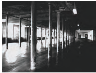
Inside of Mill # 1, Round Columns are made of wood.
