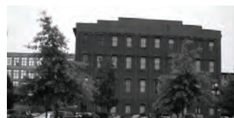
Bates Mill # 7 side view, from Lincoln Street.
