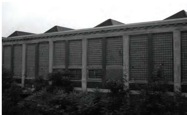
Canal side of # 5
