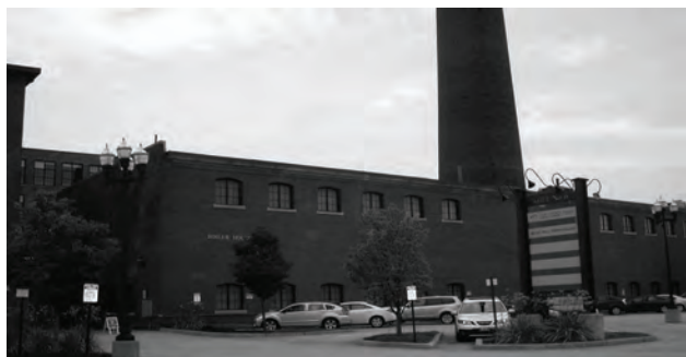
Bates # 9 Boiler House
